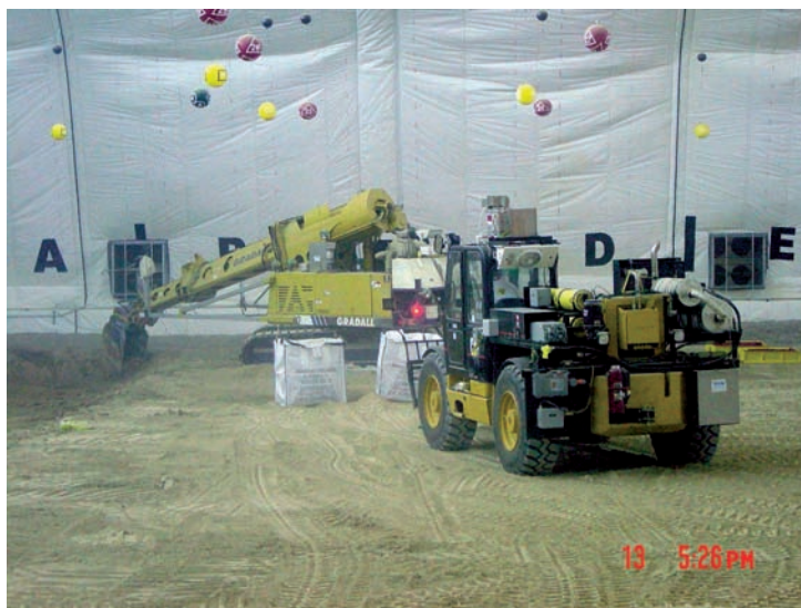
FIG. 6. Remote controlled digger.
