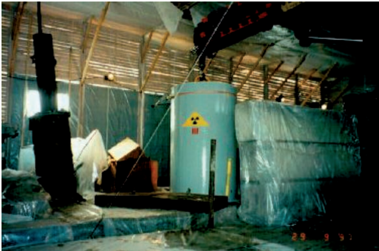
FIG. II-5. Control rod container on top of the SWR ready for transport to the interim store.
