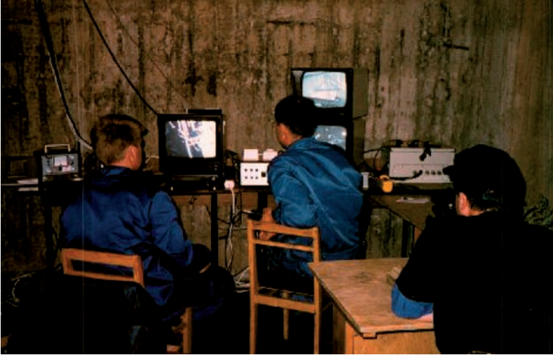
FIG. II-4. Control room for remotely controlled cranes.
